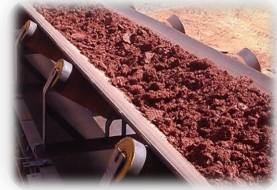
POWDER CONVEYING SYSTEM
